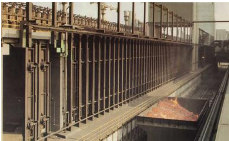
Figure 1: "Coke Side" of a By-Product Coke Oven Battery. The oven has just been "pushed" and railroad car is full of incandescent coke that will now be taken to the "quench station".
